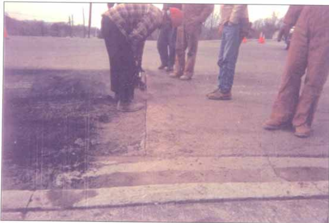
A pneumatic hammer was used to square the milled edges
