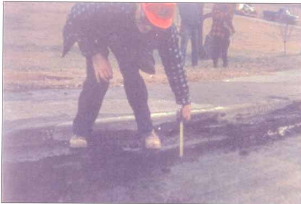
The remaining asphalt surface and gutter served as forms for the ULTRA THIN Concrete
