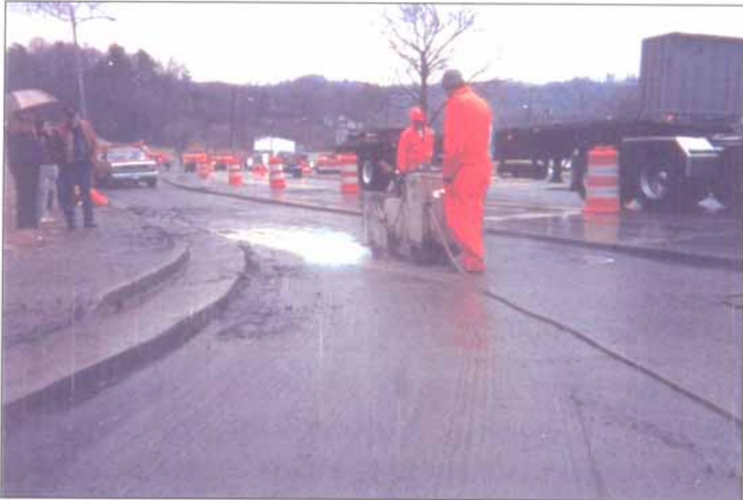
Traffic loops were cut immediately after the sweeping operation
