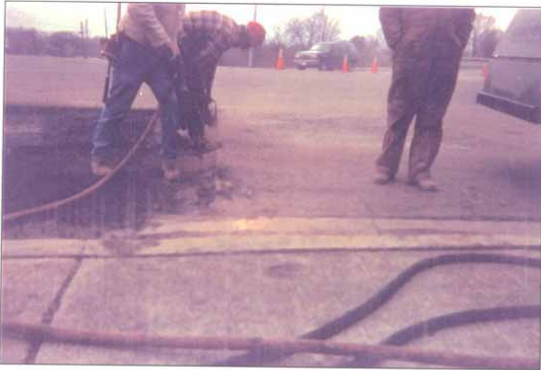
A power saw was used to get a clean, straight edge
