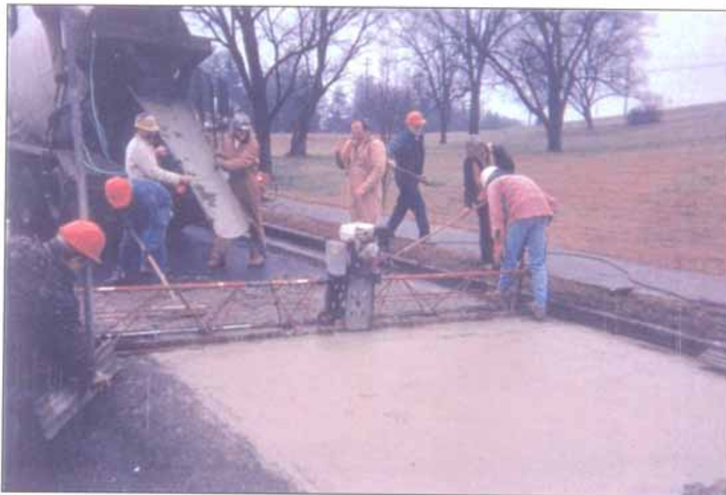
A vibrating screed was used to level the concrete
