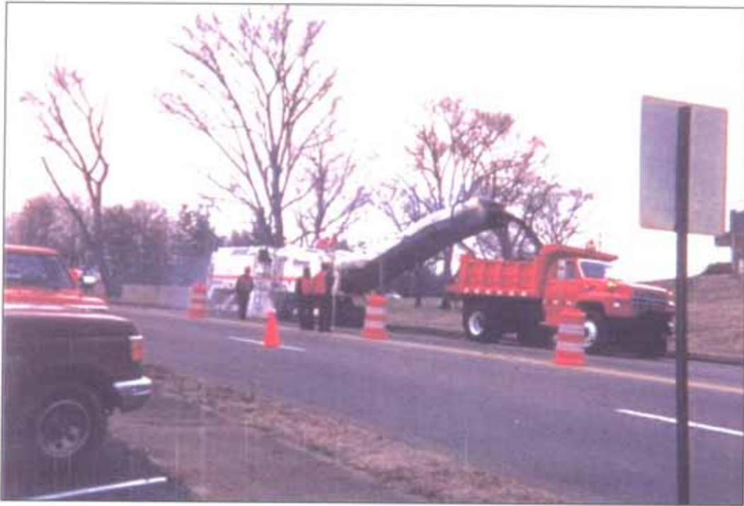
Milling to a three inch depth was done by the Tennessee D.O.T. Tuesday morning, January 11, 1994
